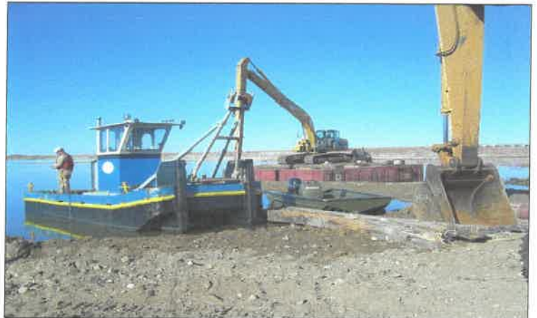
Dredging at John Martin Reservoir in 2009.
