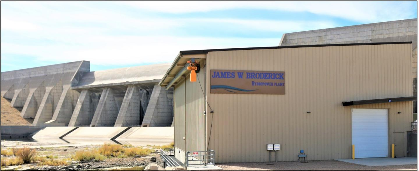
The Enterprise signed a Lease of Power Privilege with the Bureau of Reclamation in 2017, and constructed a 7.5 megawatt, \$20 million hydroelectric generation plant at Pueblo Dam. The plant was completed in May 2019. After loans are repaid, revenues will be used to offset OM&R costs of the Arkansas Valley Conduit.
