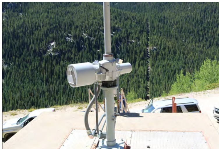
Gate actuators, such as this one at the Granite Syphon, were installed in the past few years. The remote operation reduces the time needed for Reclamation workers to travel to a site and manually open and close the gates. (SECWCD photos, 2023)
