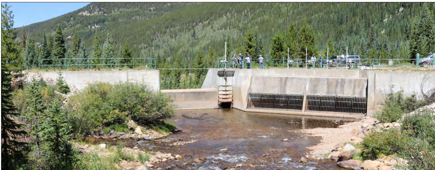
The diversion at the west portal of the Boustead Tunnel on the Fryingpan River is a key feature of the Project.
