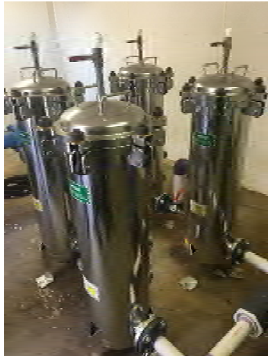
Photo 1 – Well Filtration System
