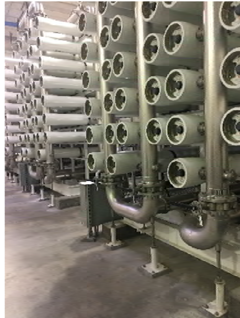
Photo 9 – 2 Stage 30 x 15 RO System
