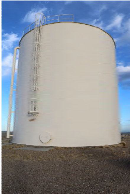
Photo 4 – Storage Tank North of Town
