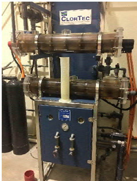
Photo 6 – On-site Hypochlorite Generator
