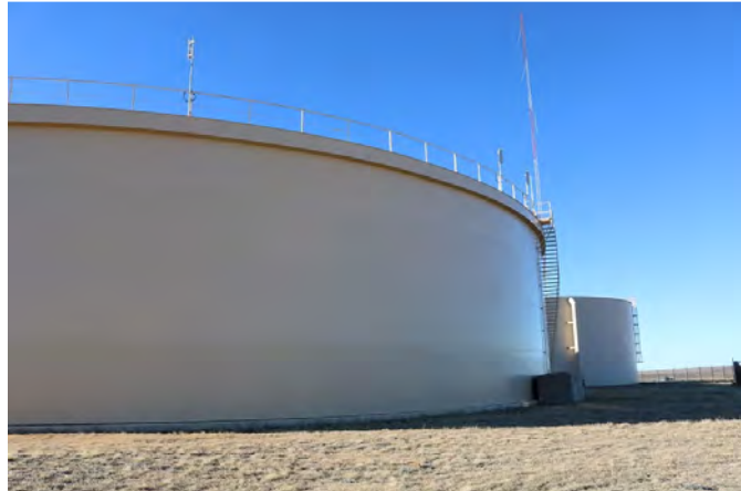
Photo 10 – Treated Water Storage Tank
