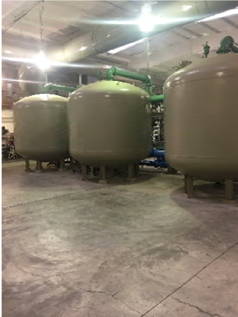
Photo 8 – Iron and Manganese Removal Filters
