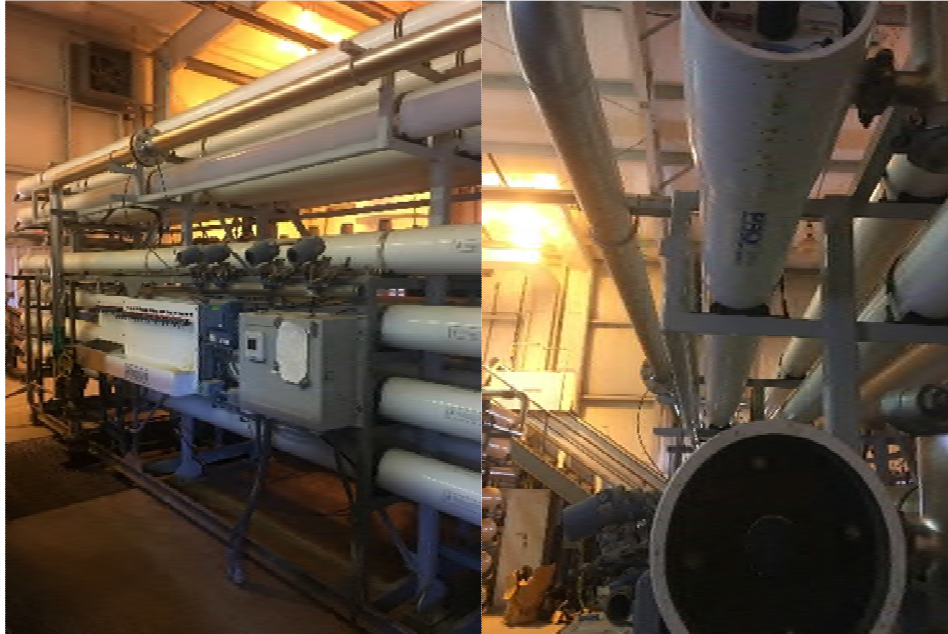
Photo 12 – RO Plant at Las Animas
