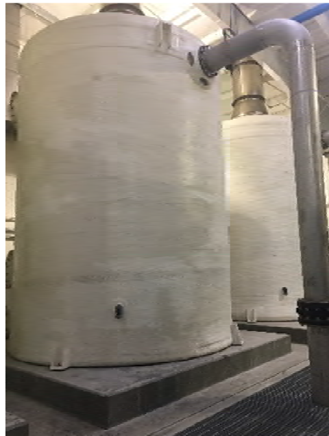
Photo 5 - RO Decarbonator
