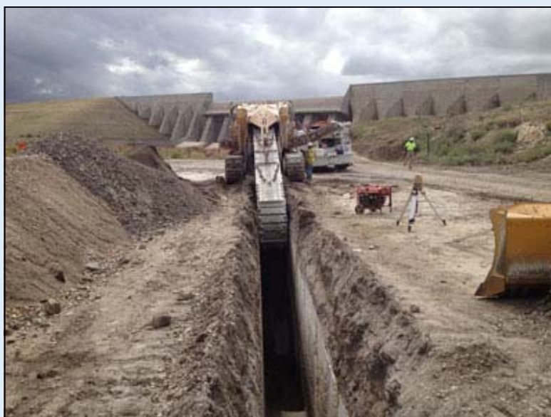
Heavy equipment digs a trench for the Southern Delivery System pipeline at Pueblo Dam.
